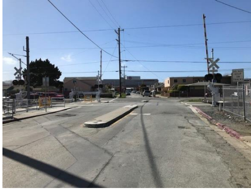
Scott Street at-grade crossing
