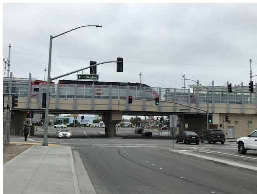
San Bruno Avenue grade separated crossing
