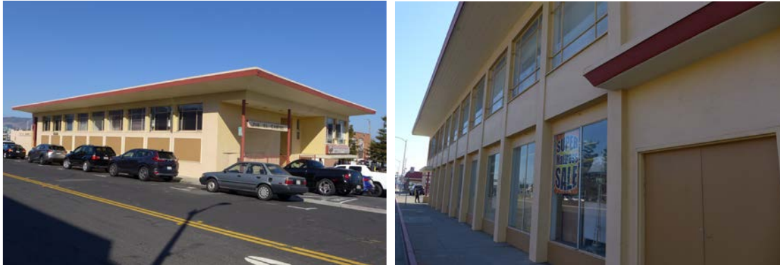
Figures 5 and 6. 715 El Camino Real, the west façade (left) and the east façade (right).
