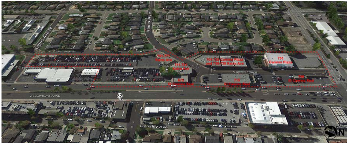
Figure 1. Aerial view of the site, the approximate boundaries of the project area outlined in red. Edited from Google Earth, retrieved November 3, 2017.
