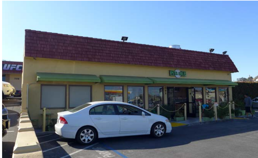
Figure 7. 799 El Camino Real, the east façade.
