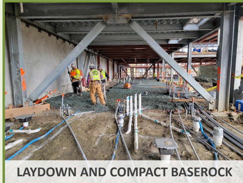
BACKFILLED TRENCHES FOR INDOOR POOL PLUMBING
