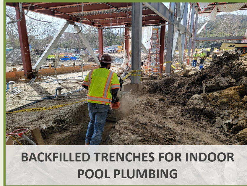
LAYDOWN AND COMPACT BASEROCK
