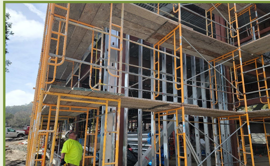
INSTALL EXTERIOR WALLS SHEATHING
