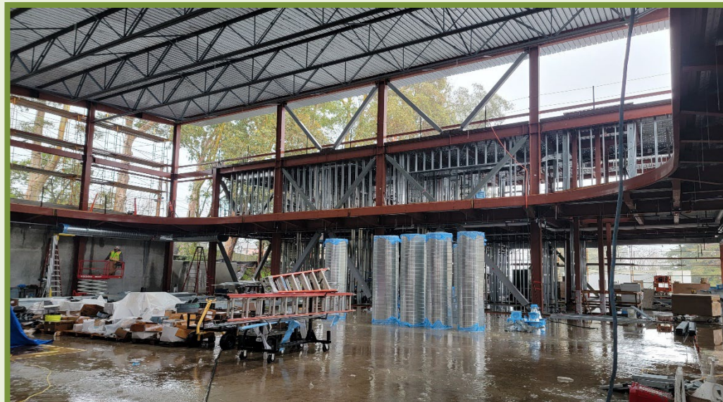
CONTINUE 1 st AND 2 ND FLOOR MEP
