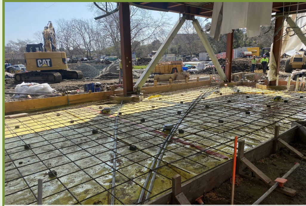
1 st FLOOR CONCRETE SLAB AT NATATORIUM
