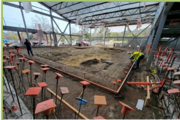
INDOOR POOL DECK GRADE AND FORMS
