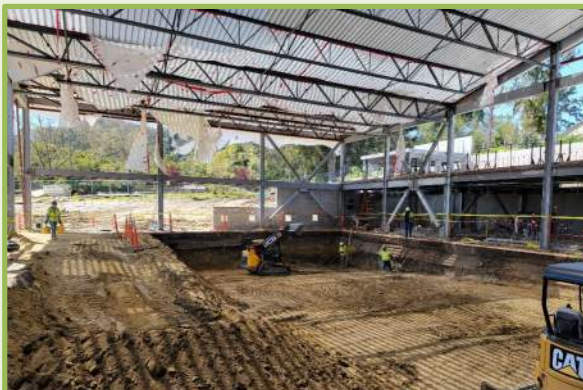
INDOOR POOL EXCAVATION
