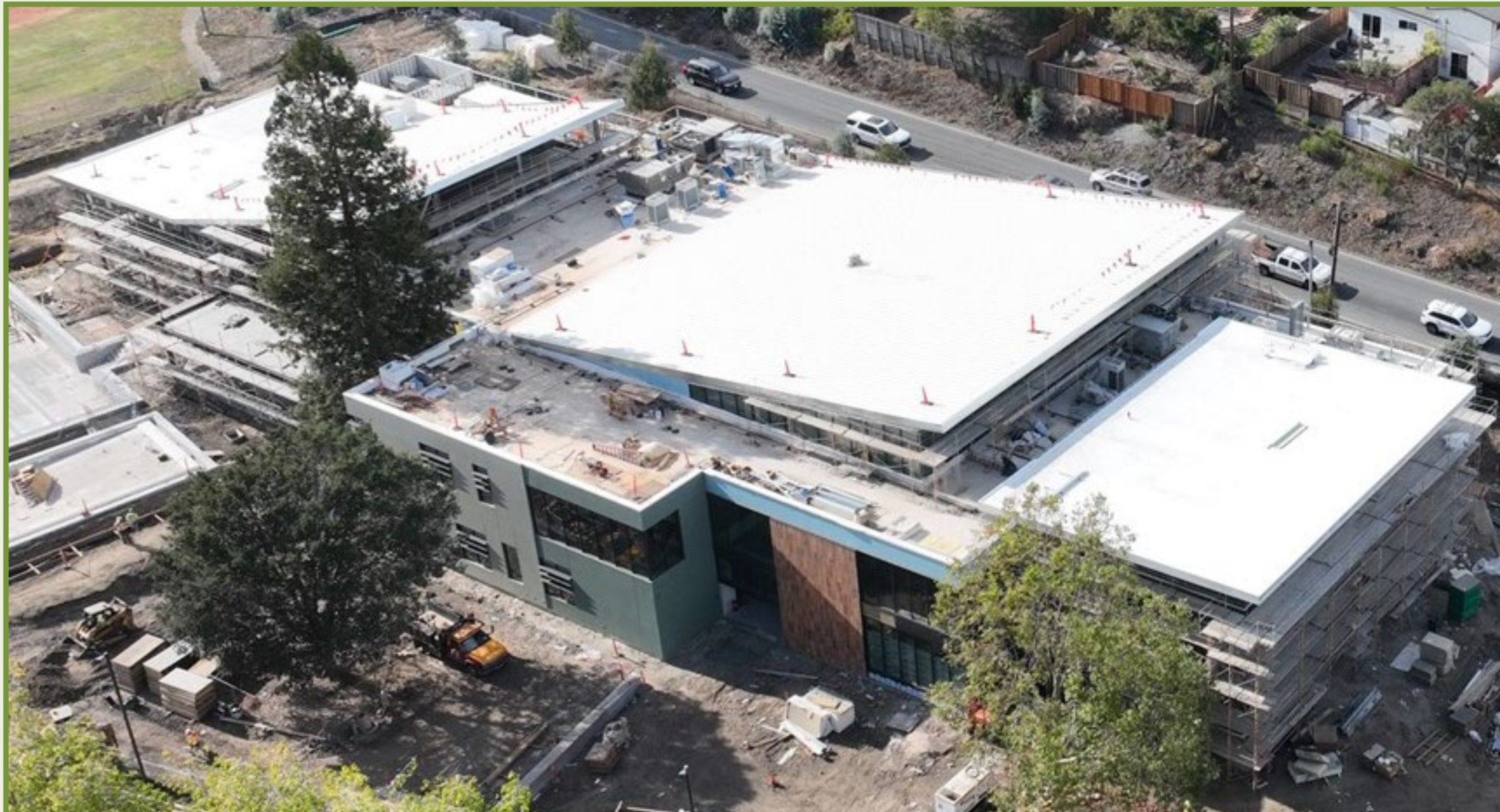
Natatorium, Gymnasium, and Community Hall Roofs
