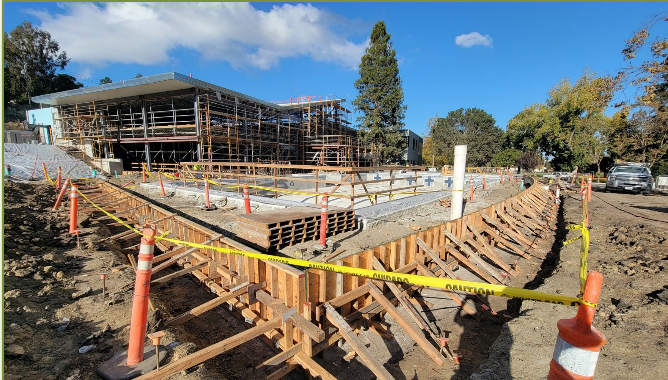
Retaining Wall and Outdoor Pools
