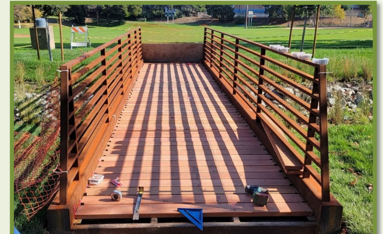
Bridge Wood Decking
