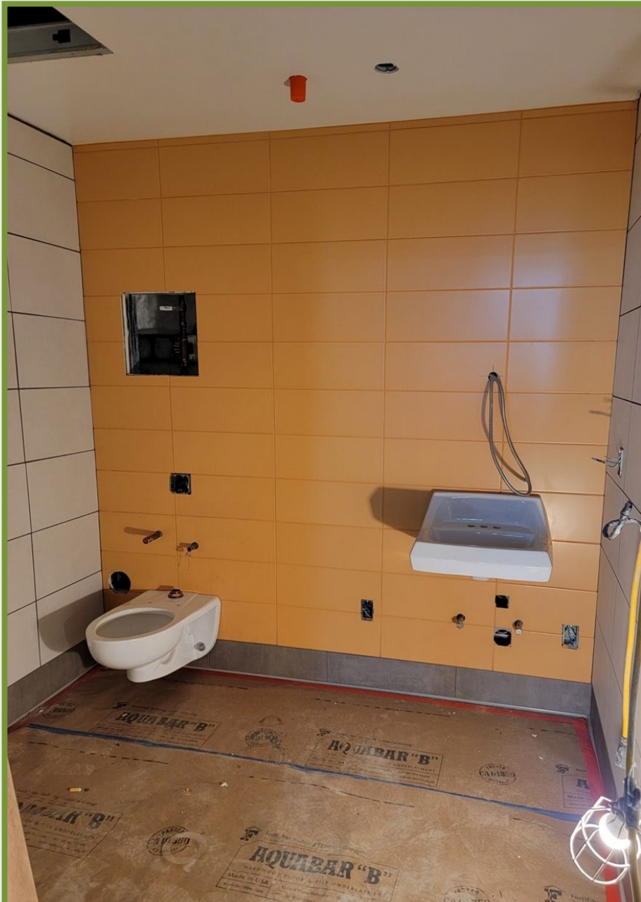
1 st Floor - Small Classroom Restroom
